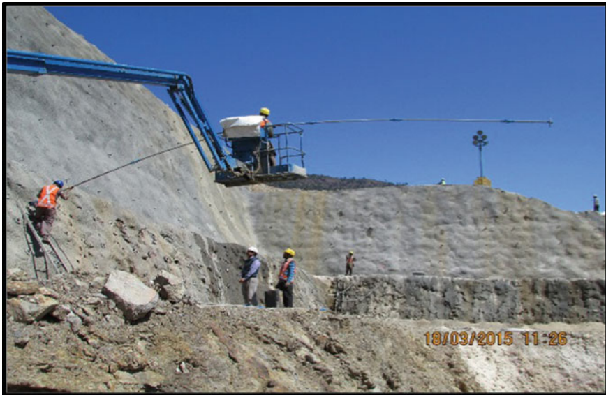
Fig. 18 Installation of rock bolts in progress
