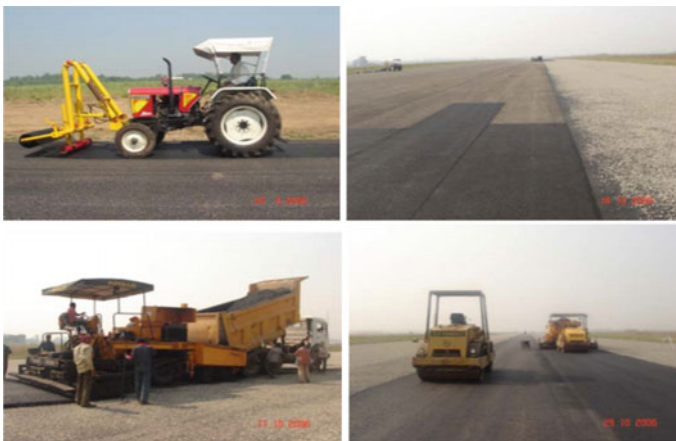
Fig. 5 Laying of glass grid, SAMI, and DBM
