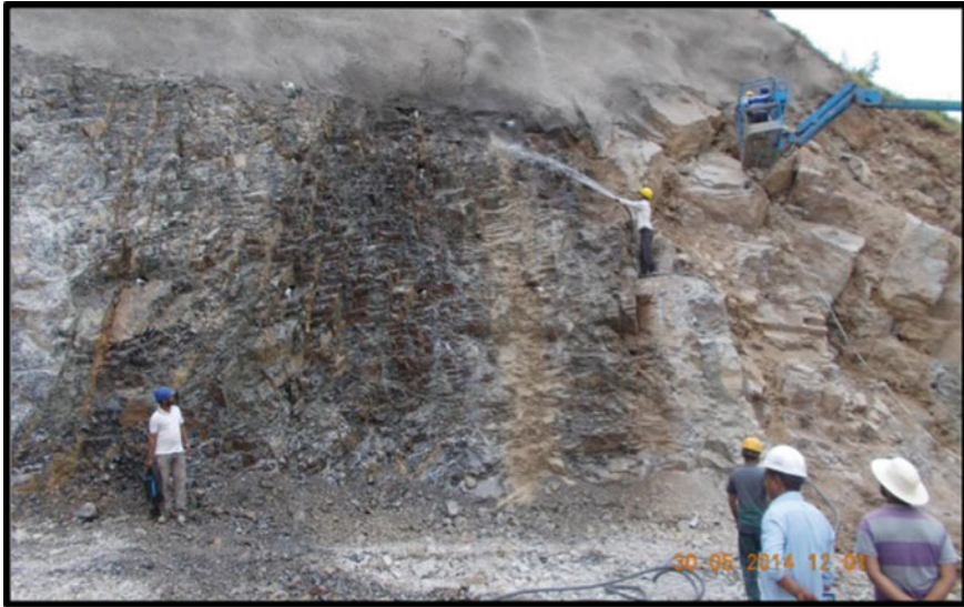
Fig. 15 Cleaning of excavated slope with water jet
