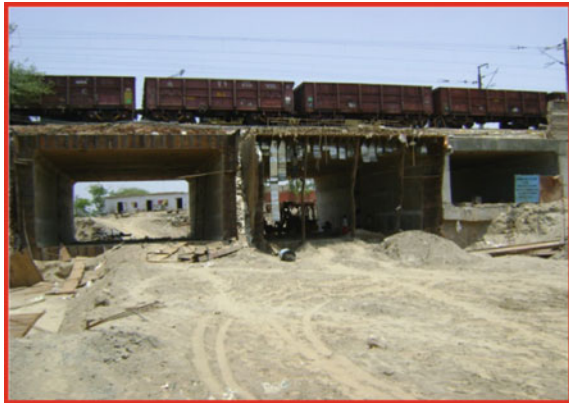
Fig. 13 GI sheet installation
