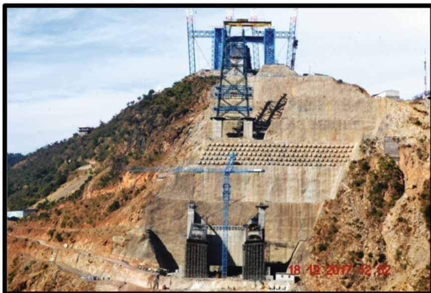
Fig. 6 Stabilized slopes on the right bank
