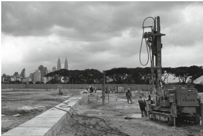
Fig. 11 Drilling rig setting up 5 m behind retaining wall
