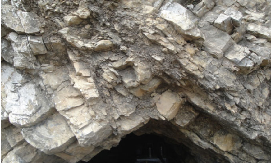
Fig. 7 Rock mass exposed at the bridge site
