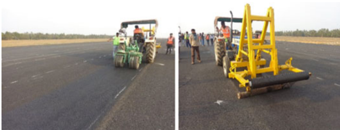
Fig. 3 Laying of glass grid
