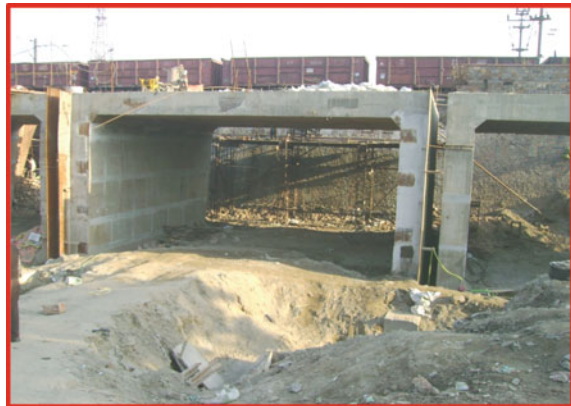
Fig. 7 Construction of boxes
