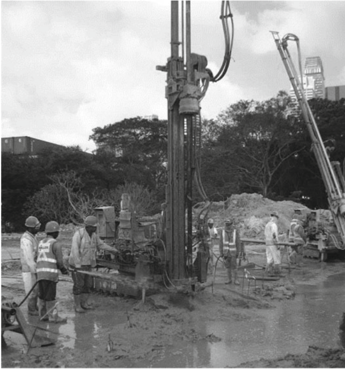
Fig. 16 Triple-fluid jet grouting
