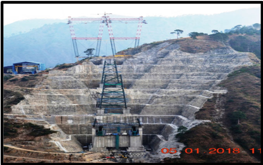
Fig. 5 Stabilized slopes on the left bank
