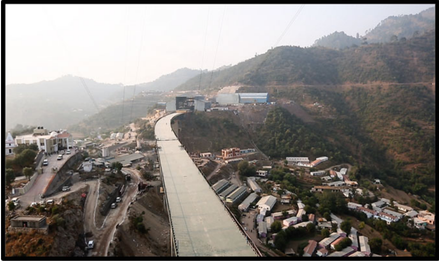
Fig. 4 Incrementally launched deck on combined circular and transition curves
